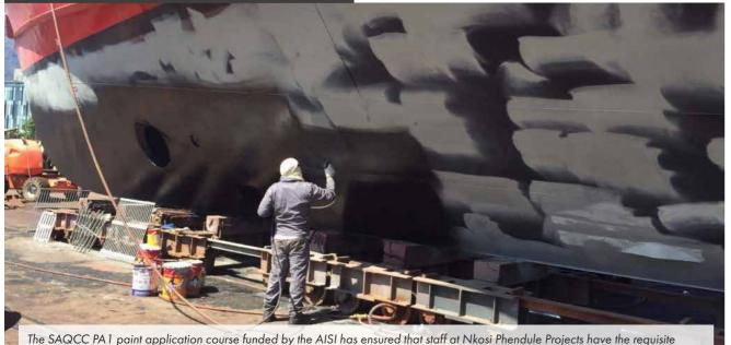
knowledge on the application of a variety of paints used in hull maintenance
