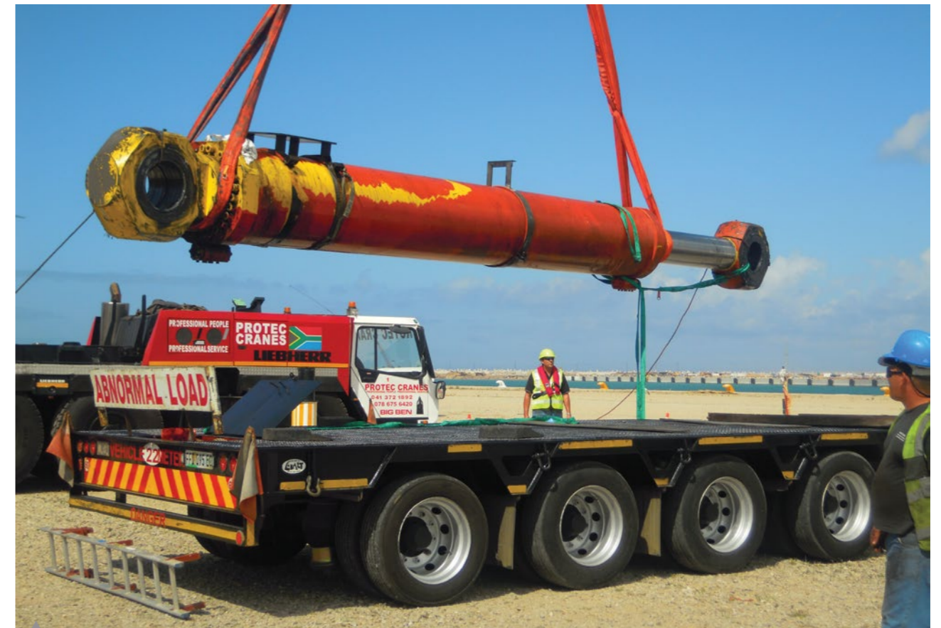
Hydraulic cylinder being removed for repair at Port of Ngqura.
