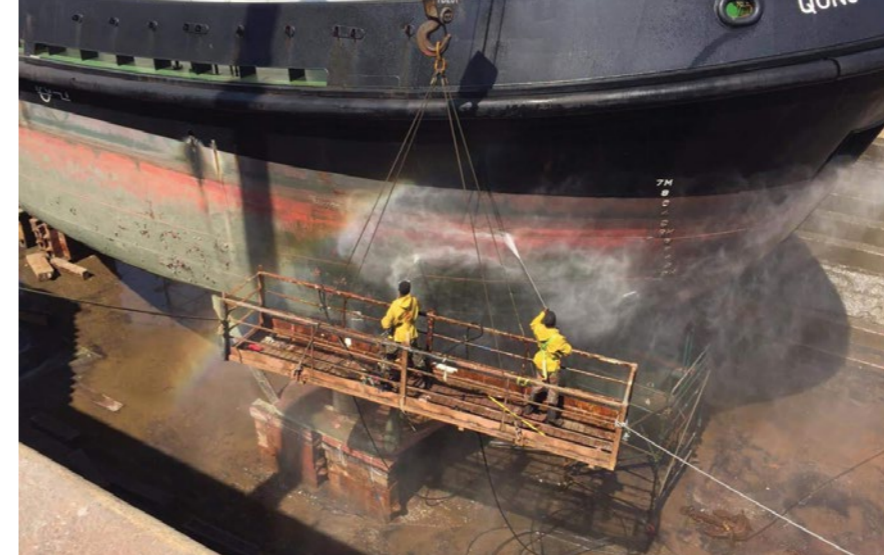
High-pressure washing to clean the hull of the tug Qunu.
