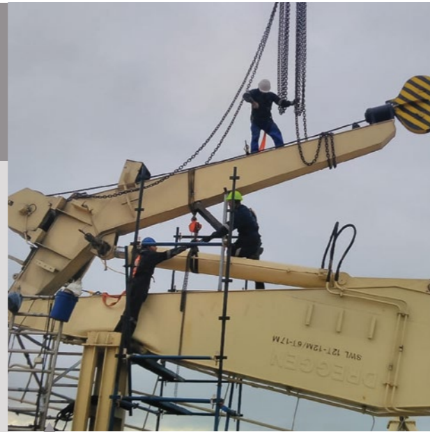
Repair of hydraulic cylinders of the knuckle boom crane.
